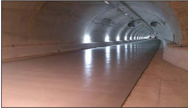
Figure 5: Concrete pavement in one of the maxilotto 1 tunnels
