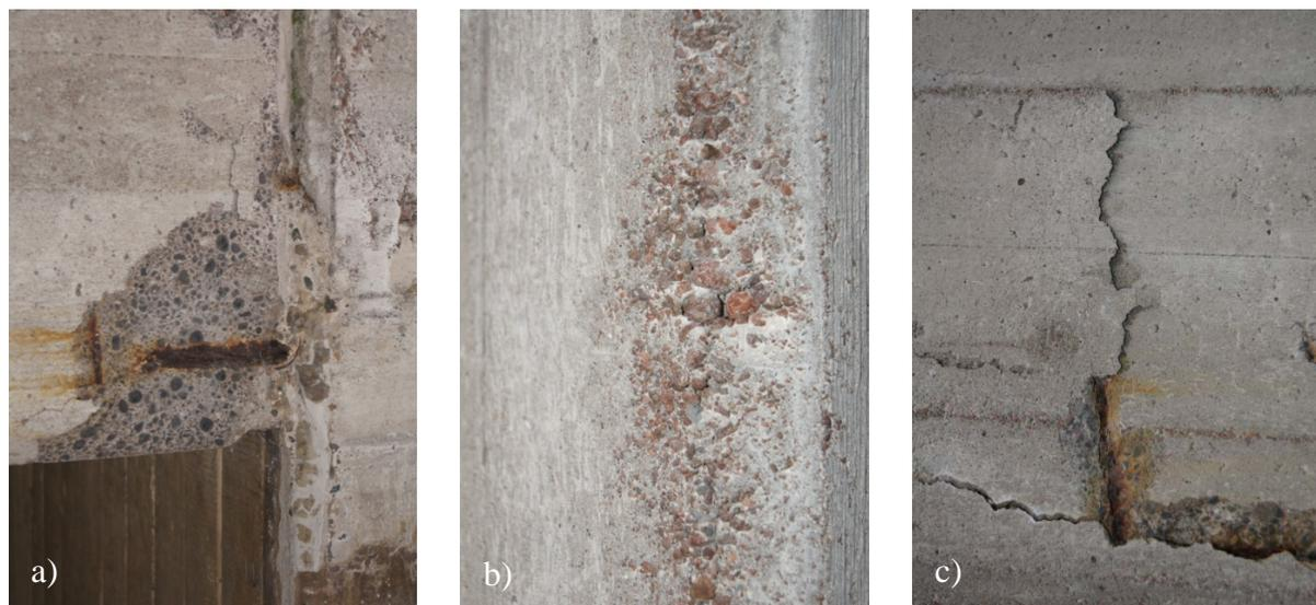
Figure 2: a) corroded reinforcement; b) rock pockets; c) cracks, spalling concrete
