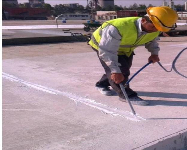
Picture 10: Cutting and curing the joints
