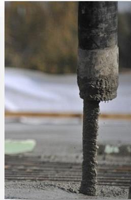
Photo 4–5: Self Compacting Concrete applied in Dominican Republic.
