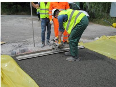
Figure 15: Mechanical compacting with vibration patch
