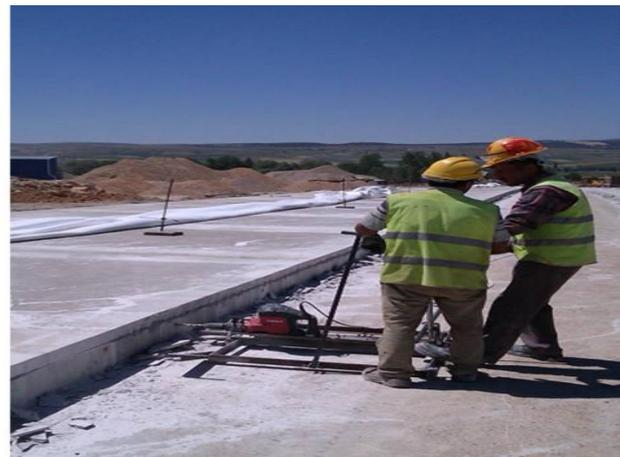
Picture 11: Curing the concrete and Tie-bar application
