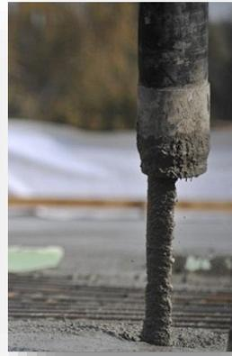
Photo 4–5: Self Compacting Concrete applied in Dominican Republic.
