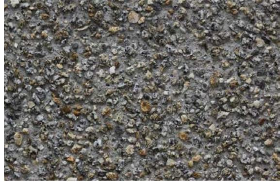
Photo 12: Washed-off surface on aggregate 2-8 mm (granite grit) and non-coloured mortar
