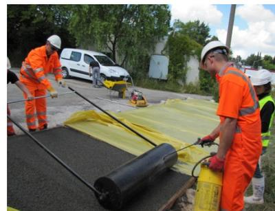
Figure 16: Compacting with hand-roll
