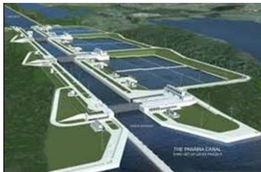
Figure 2: Proposed new locks with side water saving basins
