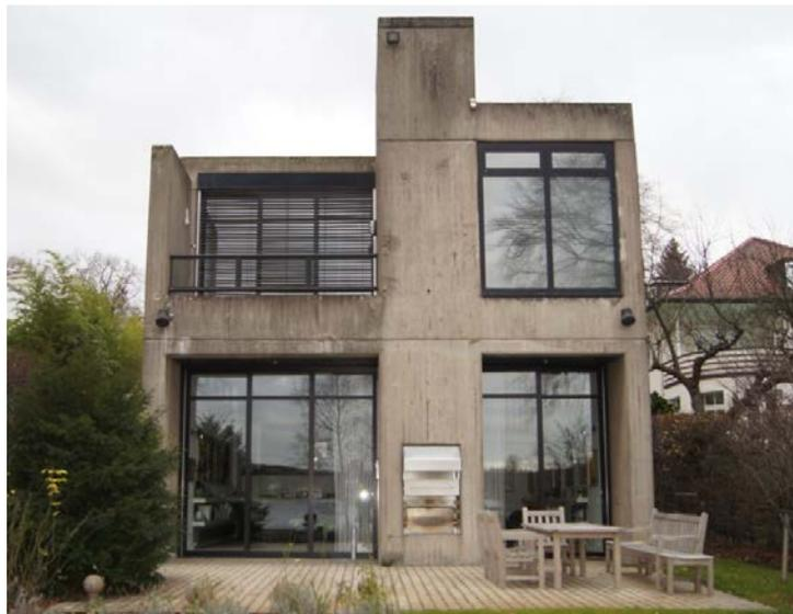
Figure1: Listed Building made of structural lightweight concrete
