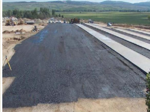
Picture 4: Protecting the sub-base from rain
