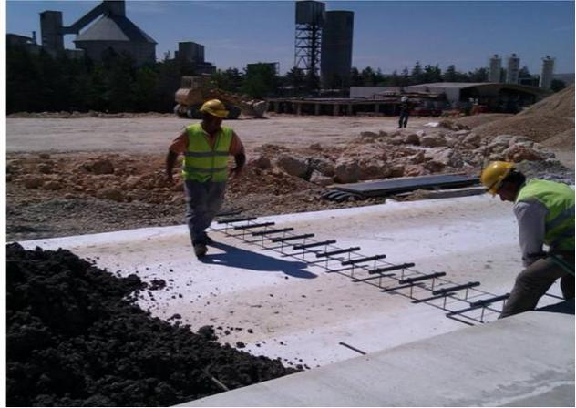
Picture 6: Spreading the geotextile and placing the Dowel bars
