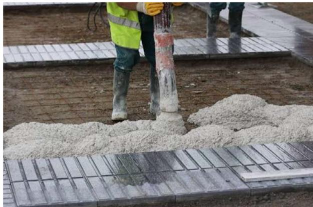
Photo 4: Pumping of concrete mix
