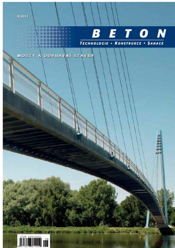
Figure 1: Example of sustainable structure footbridge in Čelákovice, near Prague, UHPC C110/130 concrete - Beton TKS magazine, issue 4/2014. (Foto J. Husák. Metrostav).
