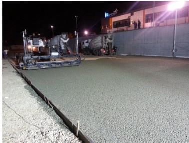
Figure 13: Placing the concrete paver
