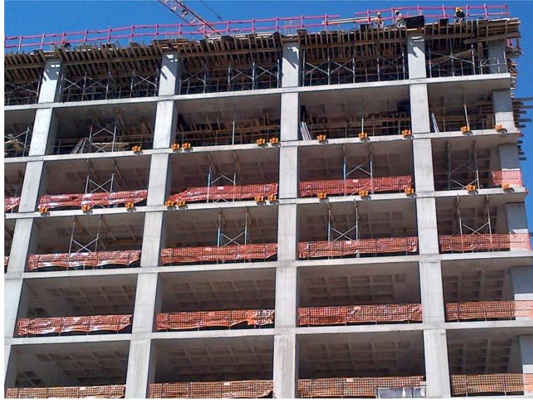
Figure 6: A typical example showing shores and re-shores for the high rise building studied.
