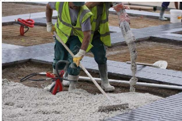
Photo 5: Spreading of mix
