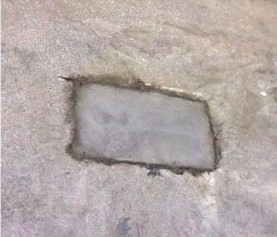
Figure 9: Repair mortar was applied to locally defective concrete surface
