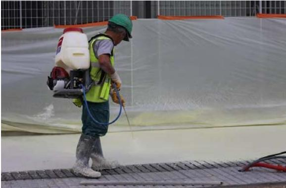
Photo 6: Spraying of deactivator
