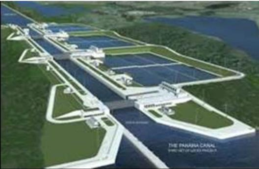
Figure 2: Proposed new locks with side water saving basins
