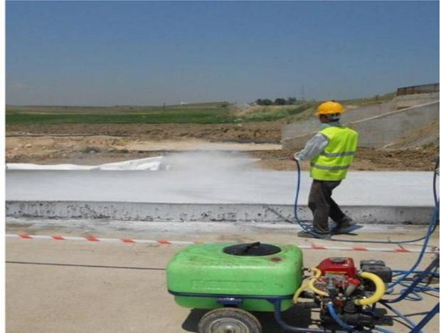
Picture 9: The appearance design and the curing of the concrete
