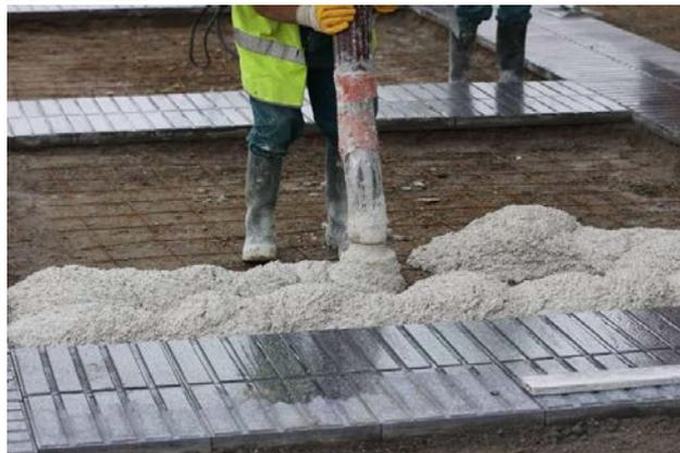
Photo 4: Pumping of concrete mix
