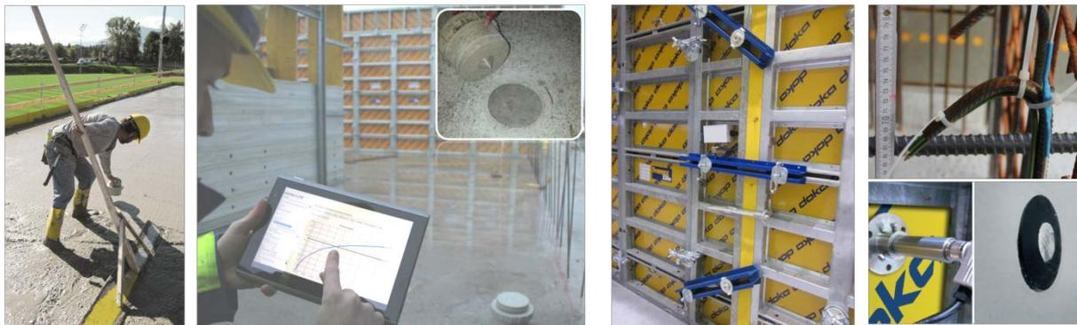
Figure2: Reusable slap sensor on the upper face of the slab and cable sensor in the wall area
