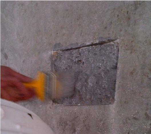
Figure 8: Application of epoxy using a brush (For strong bonding, an epoxy with two components is suggested)
