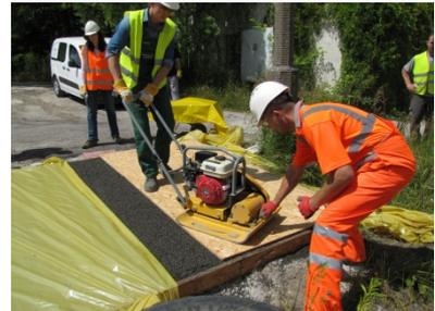
Figure 14: Mechanical compacting
