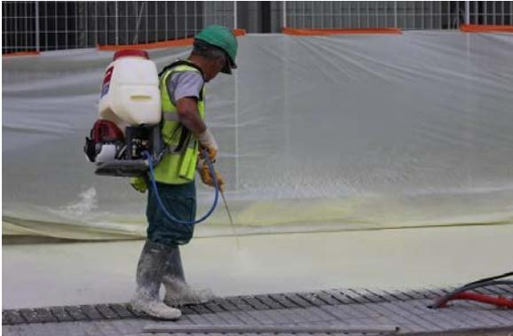
Photo 6: Spraying of deactivator
